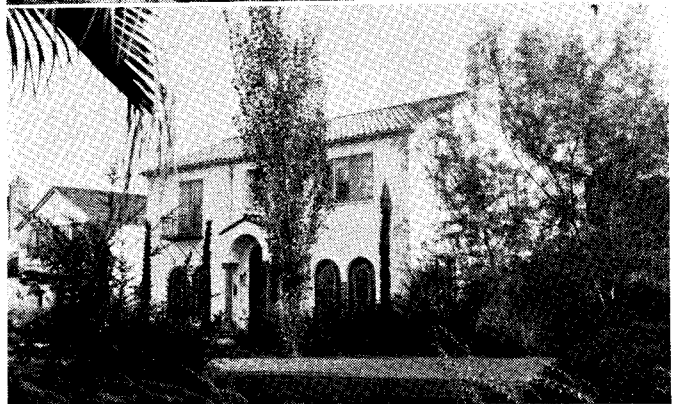
E. R. Darlington Residence, 1630 East California St., Pasadena, Calif.
