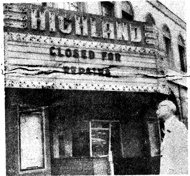
HIGHLAND TODAY — Martin Carman of Highland Park, who did a variety of jobs at the Highland as a young boy 50 years ago, looks at the "Closed for Repairs" sign on the marquee.
