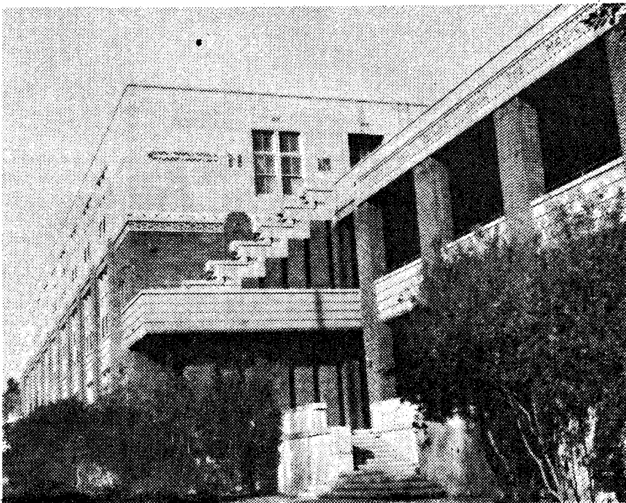
THE OLD SCHOOL —After more than 45 years of serving the Highland Park community, the familiar old brick structure was declared earthquake unsafe and demolished by the school district. Only surviving element in the new structure is the inscription honoring Luther Burbank, "Fruit and flower show the magic of his mind."
