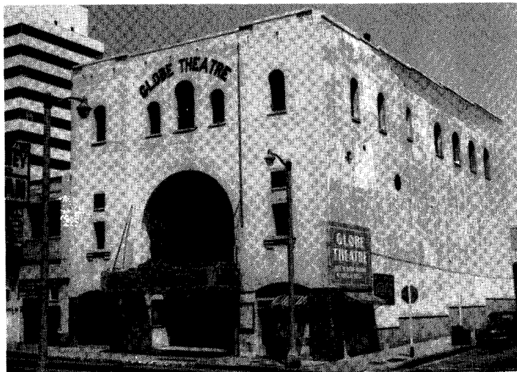
The old Globe Theatre on the northwest corner of Sixth and Palos Verdes Streets. August, 1965.
