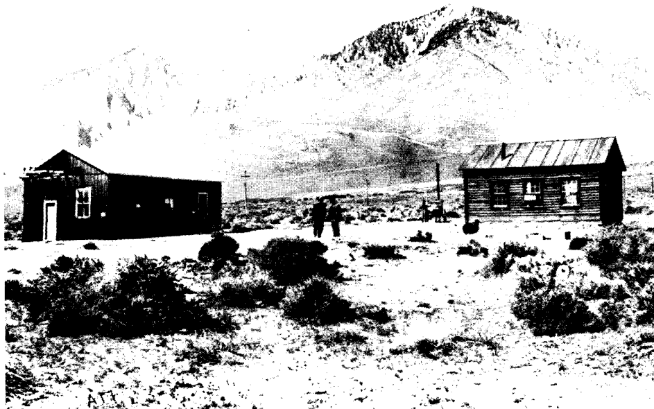
A small frame building with a tiny 120-kilowatt generator constituted the first power plant for Los Angeles, Division Creek Power Plant No. 1. Located south of Bishop, California, it began operation in 1909.
