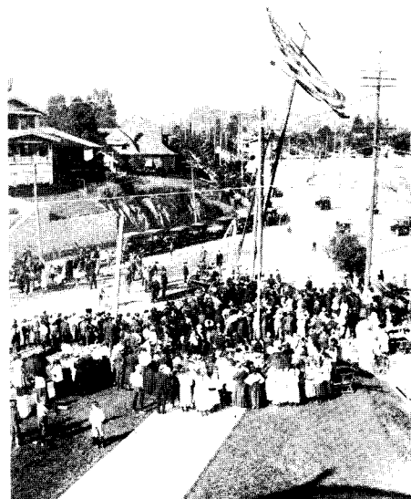
Delivery of electricity in Los Angeles began on November 13, 1916. First power pole was set at Piedmont and Pasadena Avenues.
