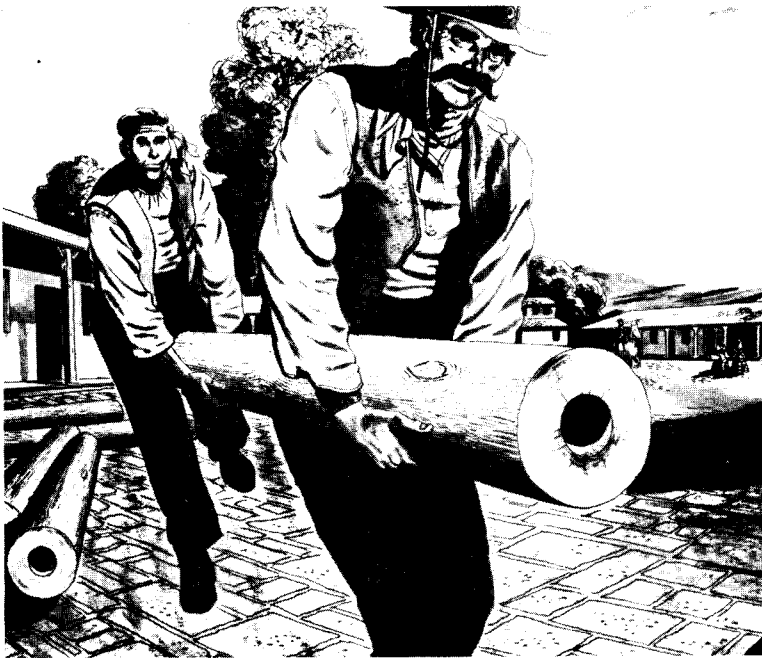
Wooden water pipes carried water to a few customers in 1857. These hollowed logs formed the first pipeline system in Los Angeles.
