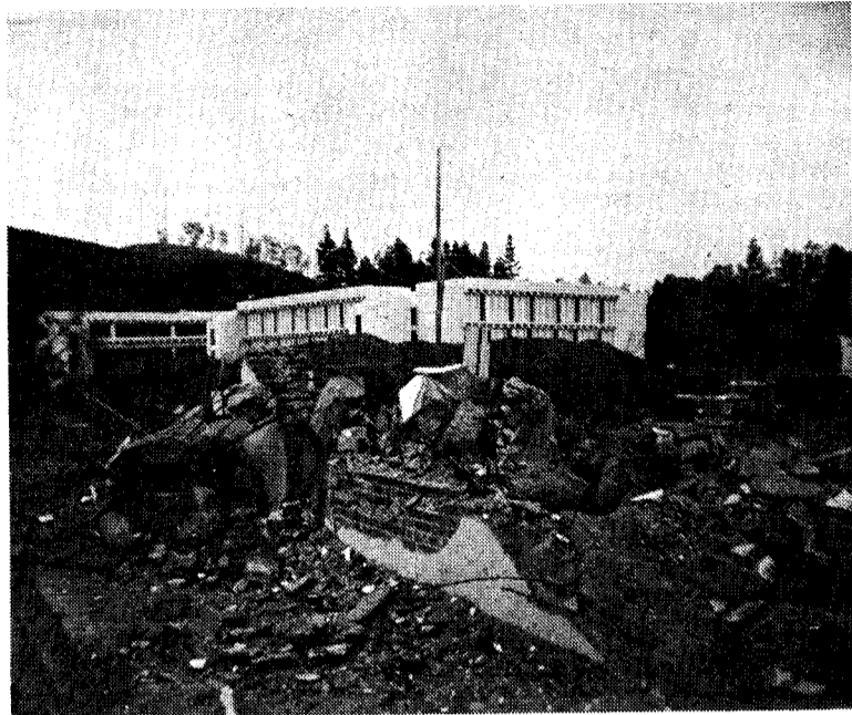
The new building in 1970 rises above the demolished original structure.
