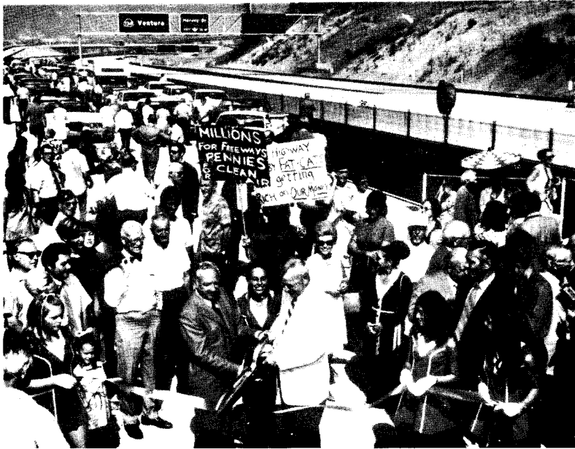
Opening at Ventura Freeway in 1971
