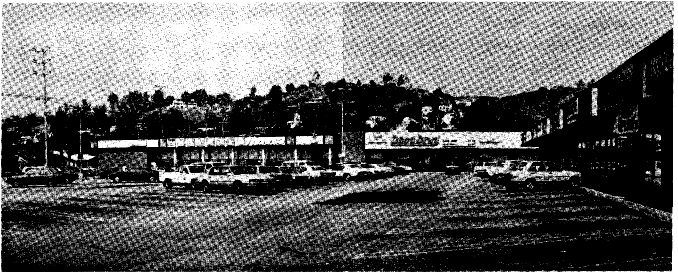
Formerly Eagle Rock Lumber Co. Now SAV - ON Shopping Plaza on Eagle Rock Blvd. at Yosemite Drive
