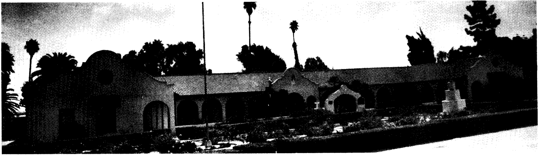
West front view of entire Domínguez Home as it appears today. The adobe portion is on the right and the 1898 addition on the left.
