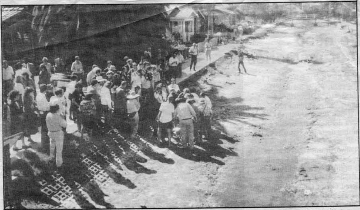
CANAL REHABILITATION — A groundbreaking ceremony for the Venice Canals rehabilitation project was held last week at Dell Avenue and Sherman Canal. (Photo by Helen O'Niell)
